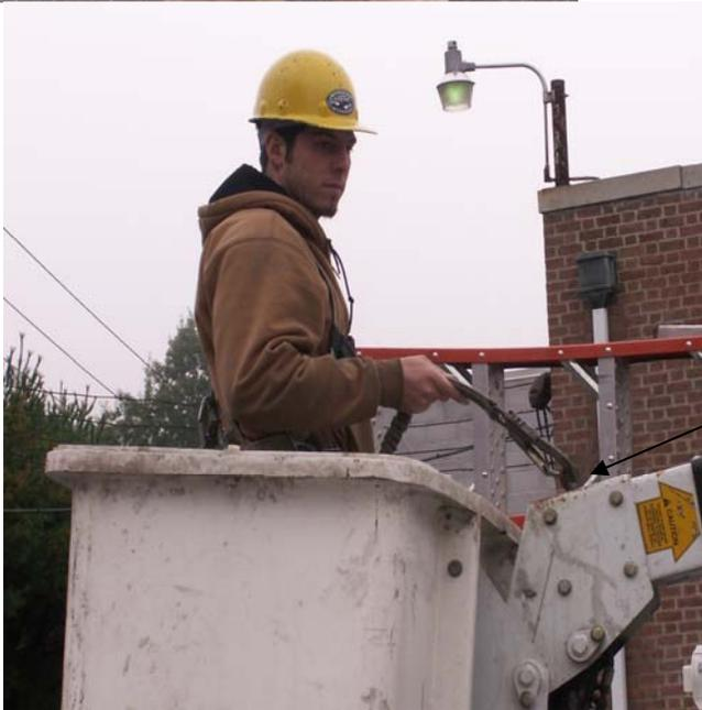
Lanyard connected to boom
